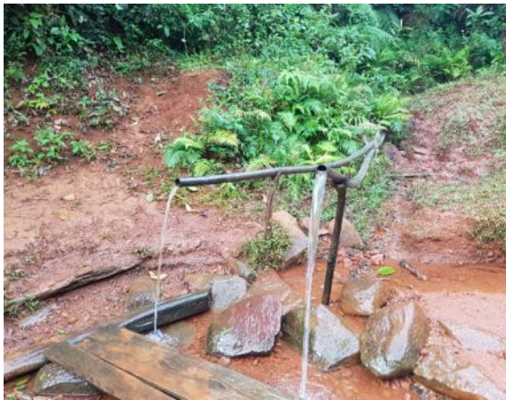
Gravity-fed water system in Xiengluang Village
